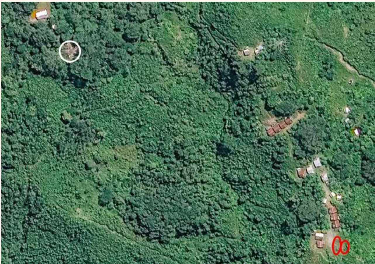
One residential house in the Lolim Village was destroyed by joint security forces after 30 September 2021. Security force personnel plundered and demolished the houses. The destroyed residential house is marked with a white circle. The village assembly hall and a neighbouring building destroyed between 13 and 29 September 2021 were marked with a red circle.
