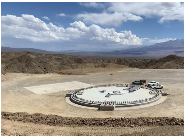
Figura 7. Finished Base Overview.
