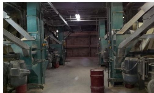
Figure 8. The environment around the equipment installing area
