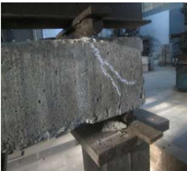
Figure 4. Failure pattern of tested SCC beams
