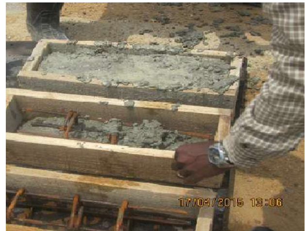
Figure 2. SCC beam specimen preparation
