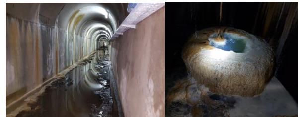
through the body of the dam.
