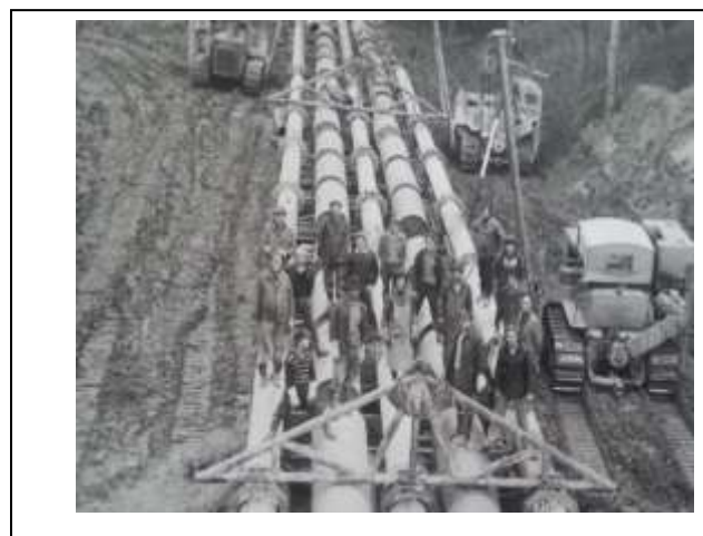
Figure 1. Danube croasing pipeline install
