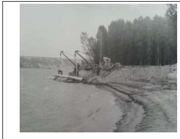
Figure 3. Danube crossing pipeline install
