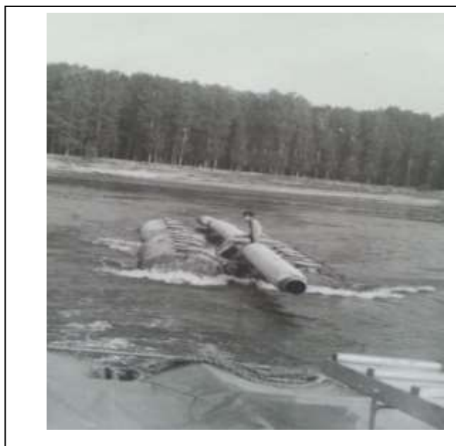
Figure 2. Danube crossing pipeline install
