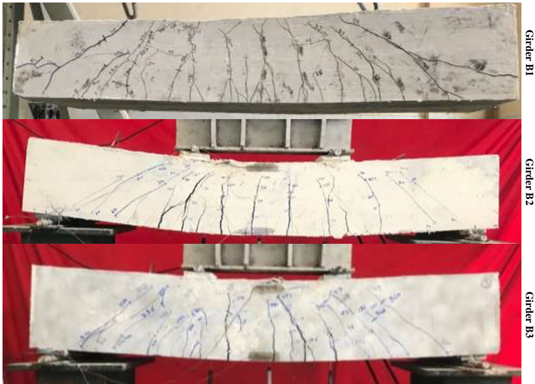
Figure 18. Cracking patterns for all tested girders.
