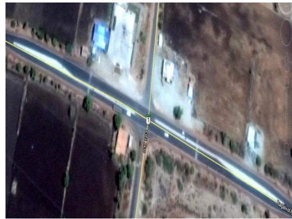
Figure 3 A cross junction provided with right turning lanes at both ends Ch 12760
