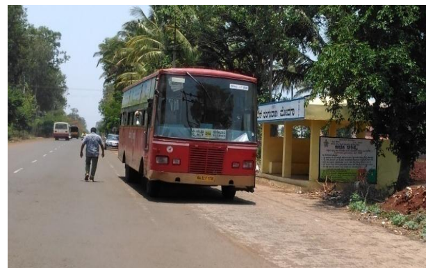
Figure 5 A bus bay and bus shelter at Ch 43257
