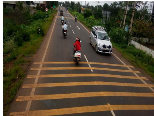
Figure 4 Transverse bar marking for traffic calming
