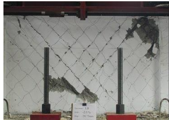
Figure 10. Cracking pattern at 2.5% drift and failure mode of specimen RL
