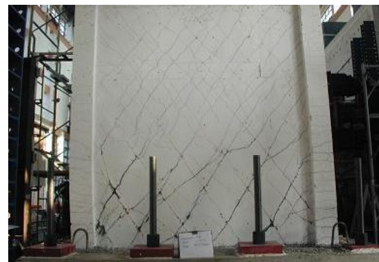
Figure 11. Cracking pattern at 1.5% drift and failure mode of Specimen RM
