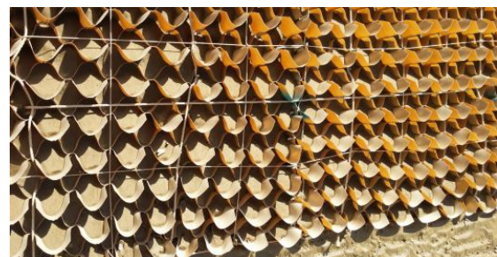
Figure 4. View of sand deposit inside coral cell and settlement of Coral cell
