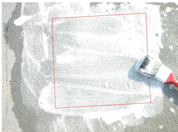
Figure 9. Cleaning of the bituminous membrane.
