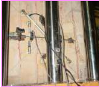
Figure 13. Cracks after compression test x direction
