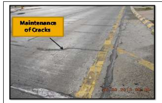
Figure # 8 ; Maintenance of cracks by crack sealing
