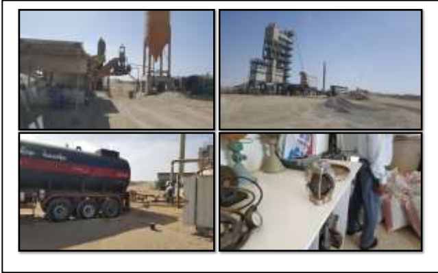
Figure # 15; Visit to asphalt batch plant
