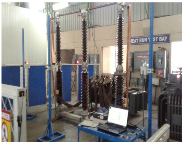
Fig. 4 Experimental arrangement for 220 kV Isolator with central break system
