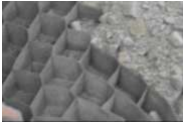
Figure 1. A view of geocell layer in the test pit
