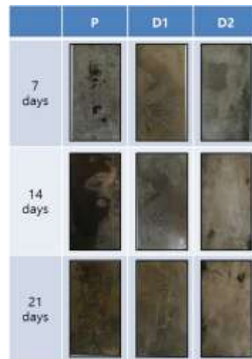
Figure 8. Steel corrosion by mix condition and age
