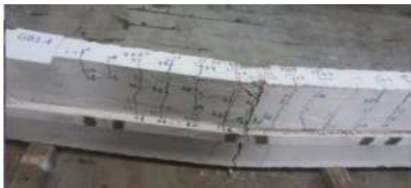
Figure (9): Shear failure of composite beam GB1.1
