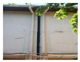
Figure 7. The separation in dilatation joints
