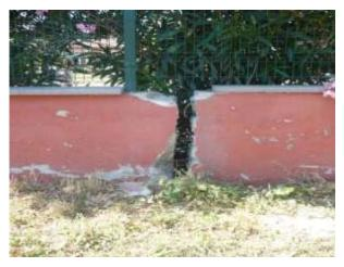
Figure 6. Seperations in walls due to soil movements
