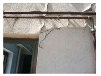
Figure 8. The cracks in column-beam connections
