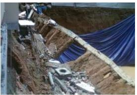
Figure 3. Trench collapse on a construction site
