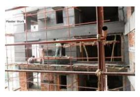
Figure 1. Workers working without any safety precaution (may cause fall accidents to the workers)
