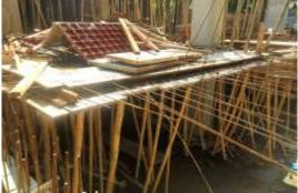
Figure 2. Bamboo props used as scaffolding and no safety net is present (may cause accidents to the pedestrians)
