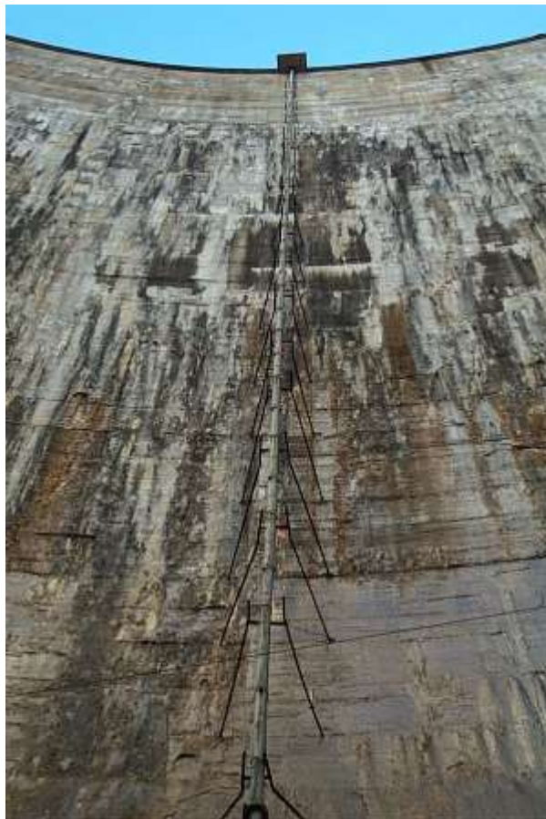
Figure 2. Pendulum in La Cohilla Dam.
