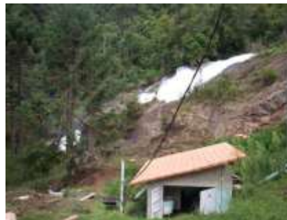
Figure 1: Waterfall and power house
