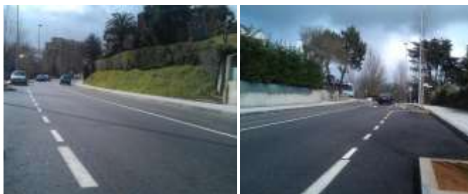
Figure 15. Road in use
