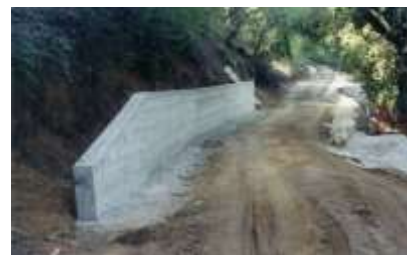
Figure 7. Concrete wall barrier.
