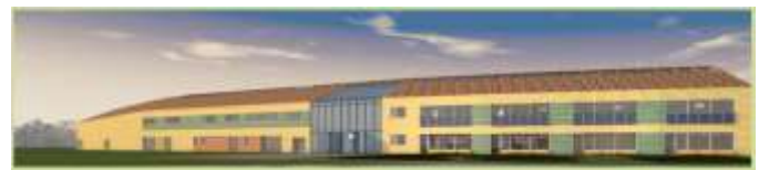
Figure 1 The school building in Dresden: compactness and high glass surface
