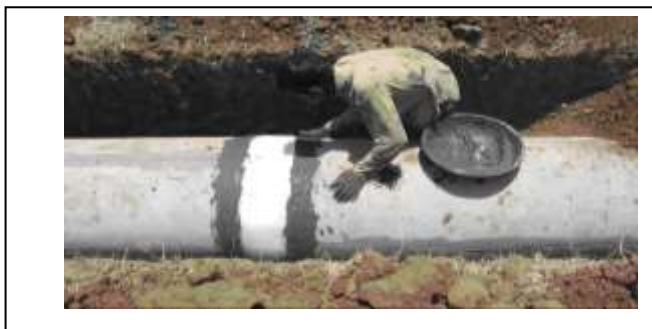
Figure 2. RCC pipes connected using geosynthetic joint
