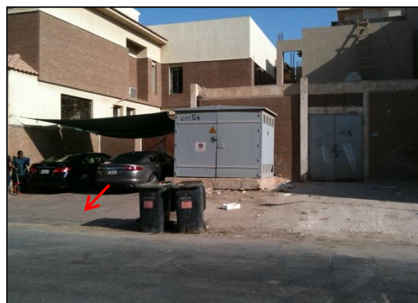
Fig. 2. Qortuba substation no. 5 indicating highest magnetic field levels.
