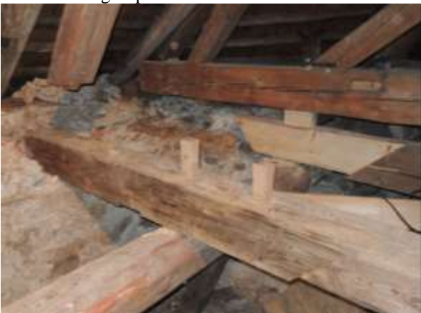
Figure 8. Reconstruction of a timber roof structure of castle in Lanškroun with help of two peg lap joint with oblique face
