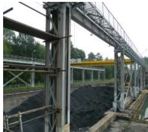
Fig. 7. View of the crane
