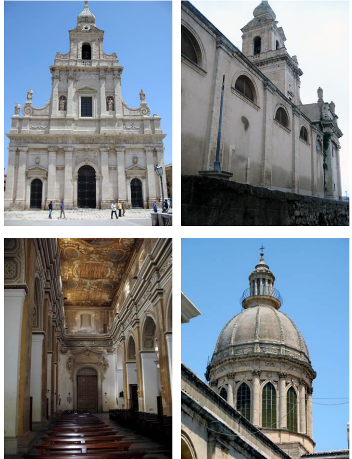
Figures 1-4. Comiso (Ragusa, Sicily), Santa Maria delle Stelle Church, external ed internal views.
