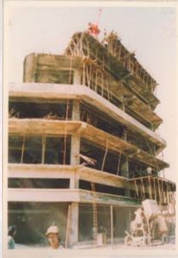
FIG.02 : EIGHT STOREYED POONAM TOWER UNDER CONSTRUCTION AT NAGPUR AND MINI CLIMBING CRANE HELPING IN LIFTING CONCRETE FROM THE MIXER PLACED ON THE GROUND.
