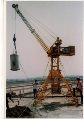
FIG.06 : HELPING BASE CONCRETING OF WALL FOUNDATION FOR COAL HANDLING PLANT AT SUPER THERMAL POWER STATION, CHANDARPUR (MS).
