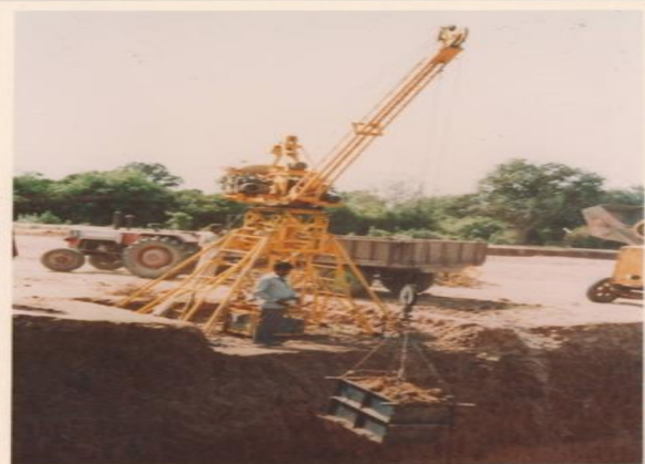
FIG.08 : MINI CLIMBING CRANE AT EXCAVATION WORK NEAR PADRA RAILWAY STATION (GUJARAT).
