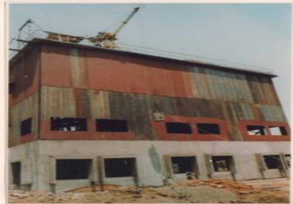
FIG.07 : MINI CLIMBING CRANE HOISTING LOAD WHILE STANDING ON THE ROOF OF THIRD STOREY.
