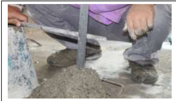
Figurer 2 Slump test
