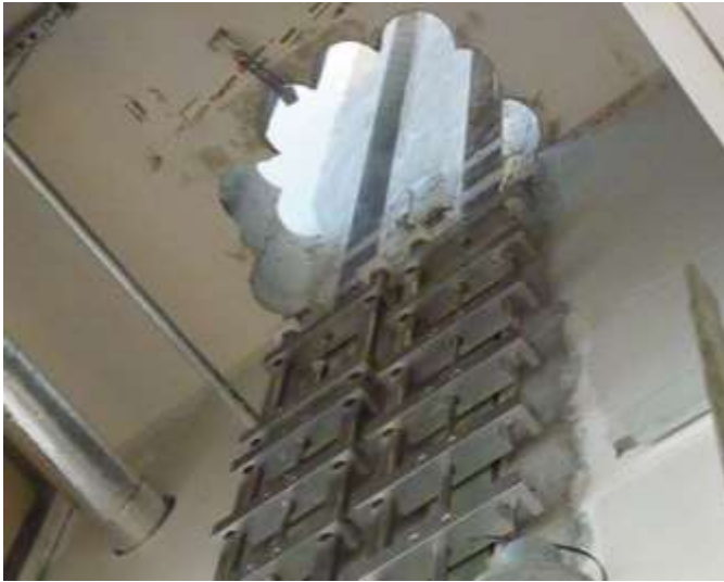
Figure 8. Strengthening of a wall in a hotel building in Sweden with four laminates, pre-stressing force of 65 kN in each laminate.
