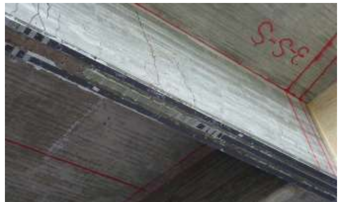
Figure 7. Strengthening of The Gruvvagen bridge in Sweden with three laminates, pre-stressing force of 110 kN in each laminate.
