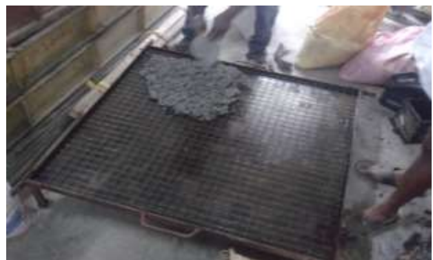
Figure 3. Casting of Reinforced Geopolymer concrete slab and conventional RCC slab
